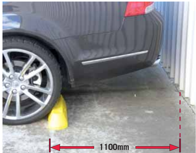
Rear into a high kerb or wall.
